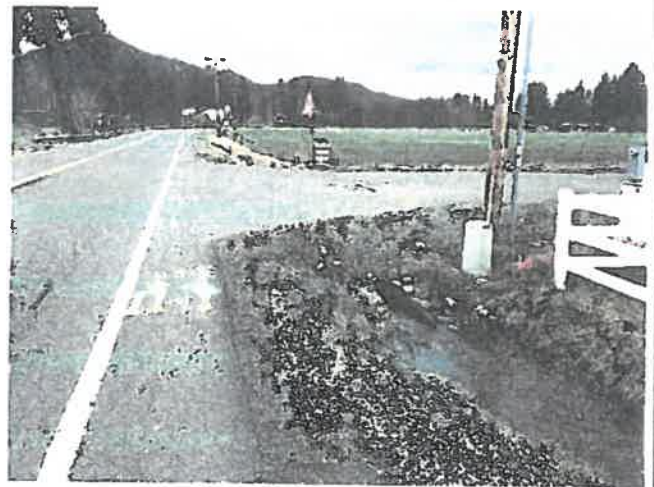
Paved Apron from Nelson Siding to Big Creek Rd
