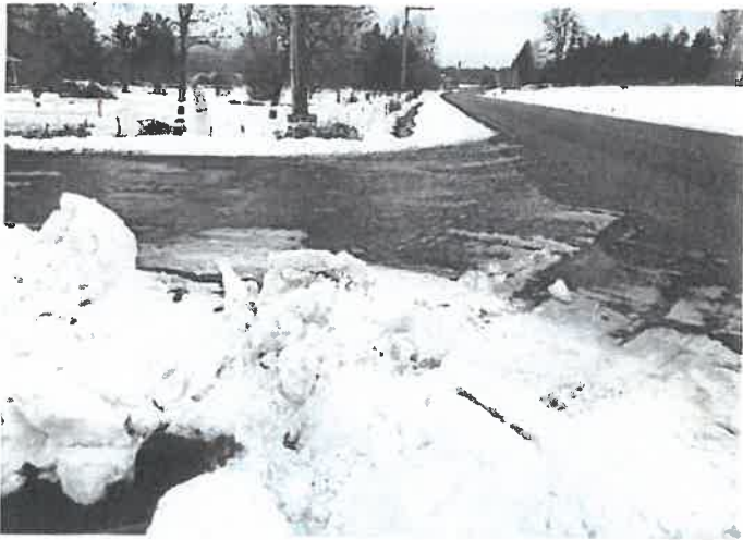
Looking east at culvert & paved access off Nelson Siding
