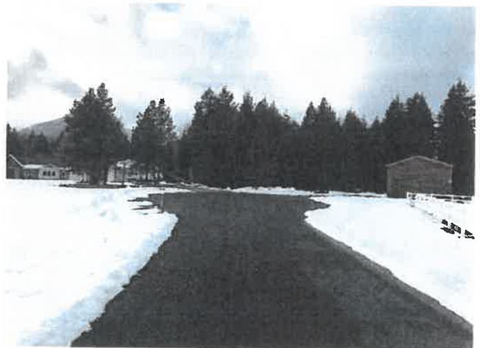
Looking west at the turn-around
