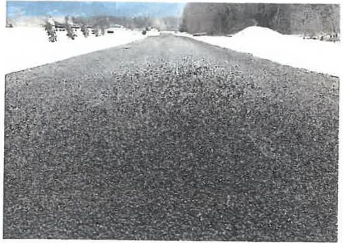
Looking south along Big Creek Rd
